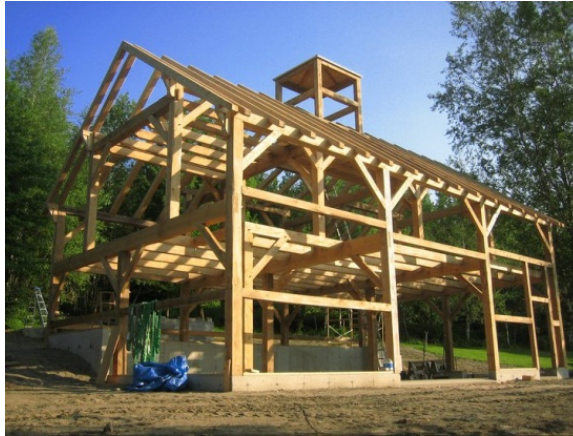
Figure 3.1: Exposed timber frame structure in Jay, Vermont, looking south-west
