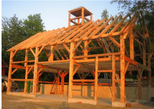
Figure 2.3: Exposed timber frame structure in Jay, Vermont, looking north-west
