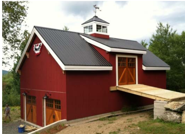
Figure 2.4: Completed timber frame structure in Jay, Vermont, looking north-east
