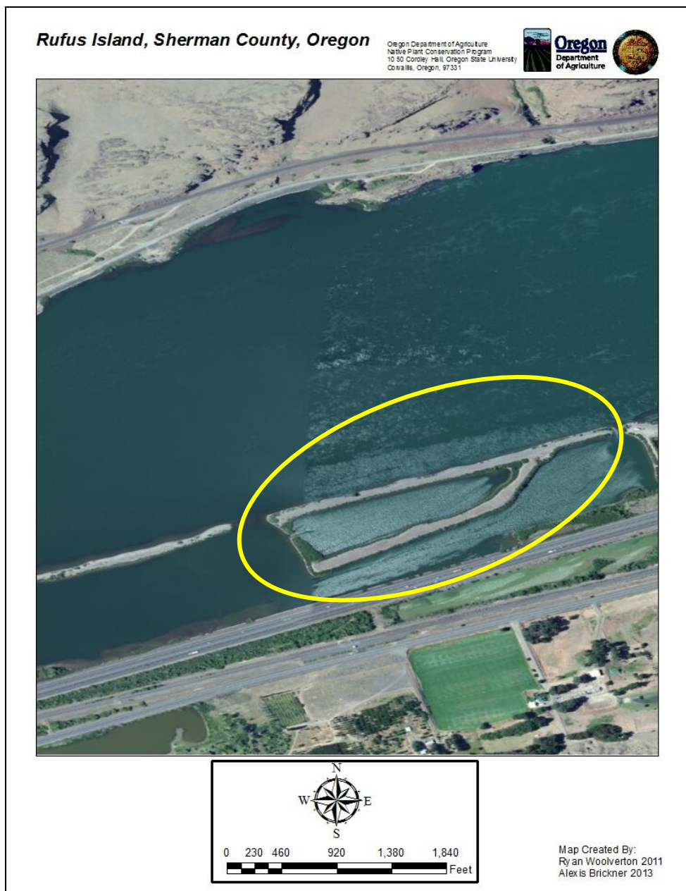
Figure 3.1. Rufus Island (see yellow circle). is located approximately 5 miles west of the town of Rufus, OR. It is part of a series of cobble bars created during dam construction. Interstate-84 runs adjacent to the island.
