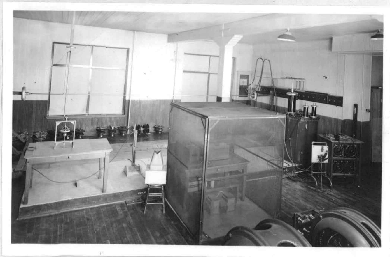
FIG.3 LABORATORY APPARATUS FOR DETERMINING POLARITY CHARACTERISTICS OF 6.25-cm. SPHERE-GAP.
