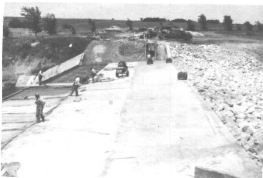
FIG. XII. A FEW SPILLWAYS HAVE BEEN RAISED
