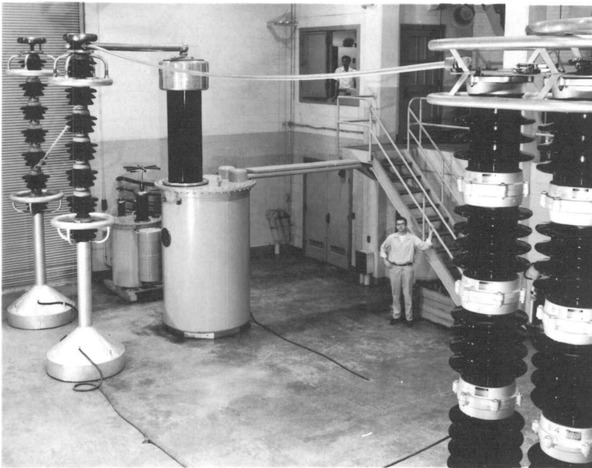
Figure 19. High-voltage laboratory showing 350 kv transformer and insulator pedestal, in left background.
