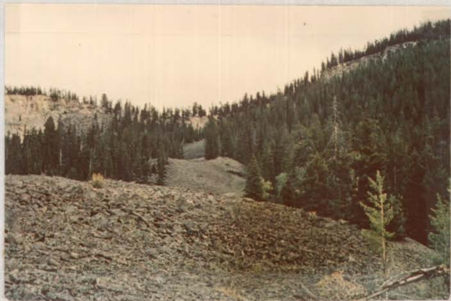
Figure 24. Taylor Fork rockslide. View looking southeast up to the headwall of the slide.
