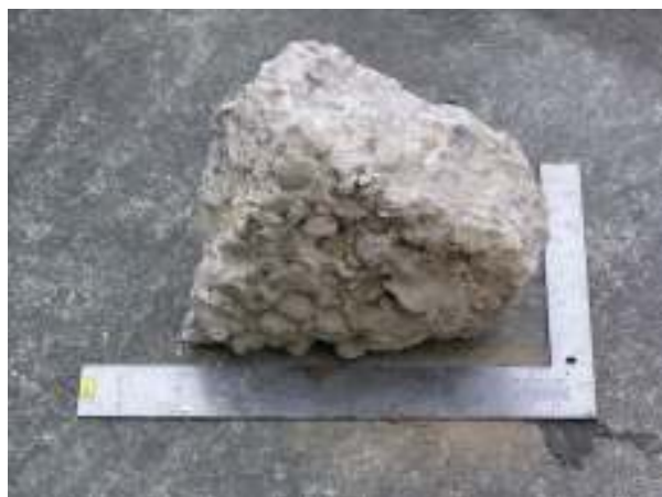
Figure 4.1 Old Concrete Prior to Cut
