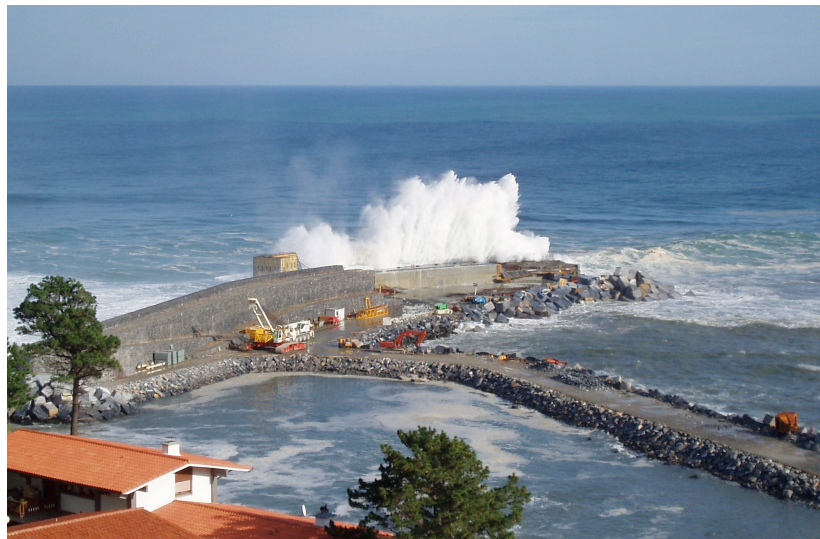
Fig. 1.5. Mutriku Breakwater, Spain 2008: water flowing through the turbine holes of the OWC. Photo credits: Félix Azpiazo.
