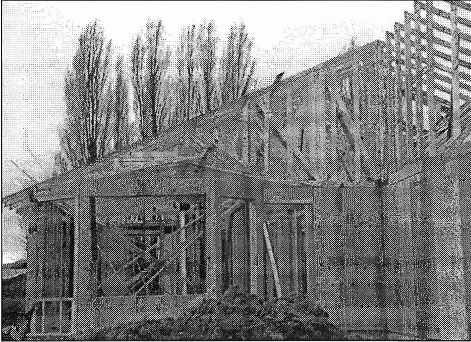
Figure 1-1. Typical Residential Construction using MPC Joints.
