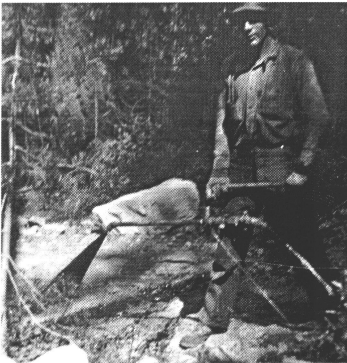
Figure 1. Hand oiling of the trail to Sperry Chalet, ca. 1932. Photo courtesy Glacier NP archives.
