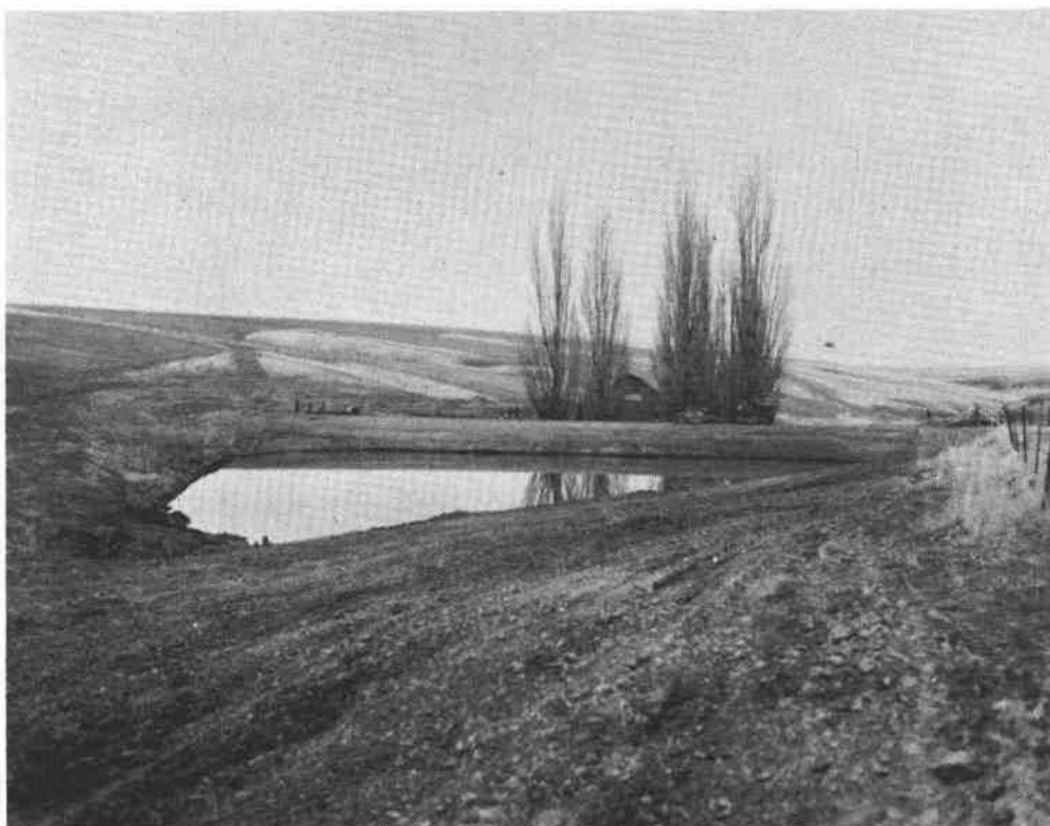
Figure 26 A typical combination earthfill and excavated stockpond nearing completion in sub-basin 3.
