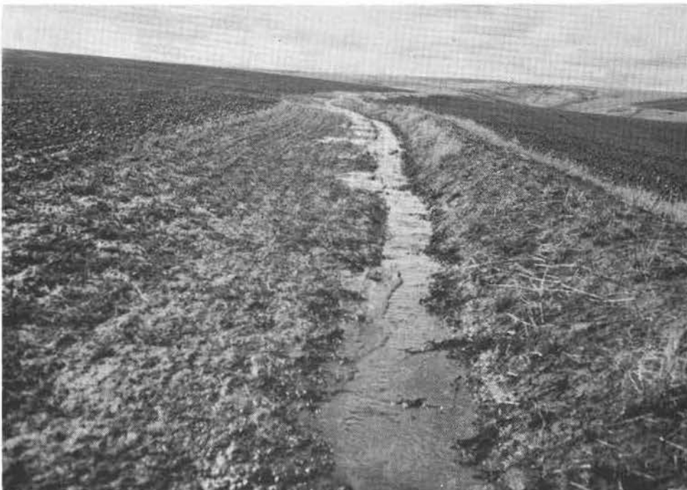
Figure 25 Controlled evacuation of runoff water by use of a contoured field diversion, sub-basin 3.
