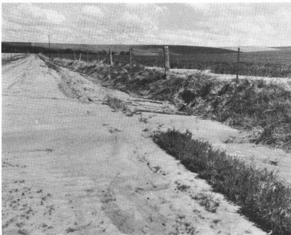
Figure 16 Siltation of Gilliam County road by sediment from wheat field, 1961.
