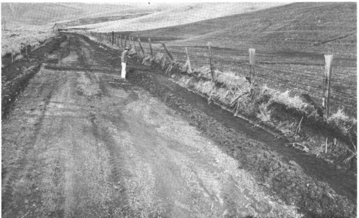
Photo 26.--Topsoil has been graded off a market road like snow in the Wasco Resource Area, Oregon. SCS photo. NO. 7-1091-5
