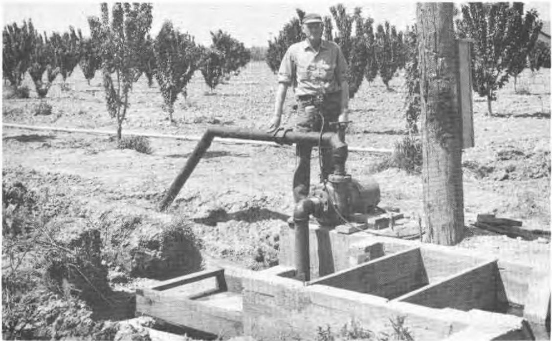
Figure 34.--This structure screens out weed seeds and some silt from irrigation water in subbasin 1. SCS photo. 7-1116-7
