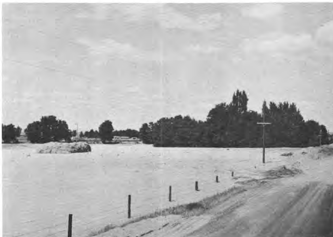
Figure 24.--Sedimentation damage to crops, land, fences, utilities, and roads resulting from a break in a canal in subbasin 2. SCS photo. 7-253-11
