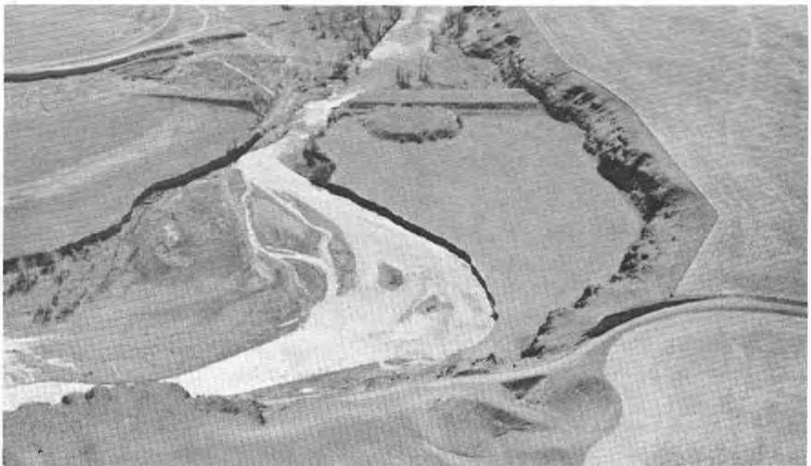
Figure 31.--Furnish Reservoir was abandoned due to sediment after 22 years. Alluvial fill in the old reservoir is now being cropped and in turn eroded away by the Umatilla River, subbasin 2. SCS photo.
