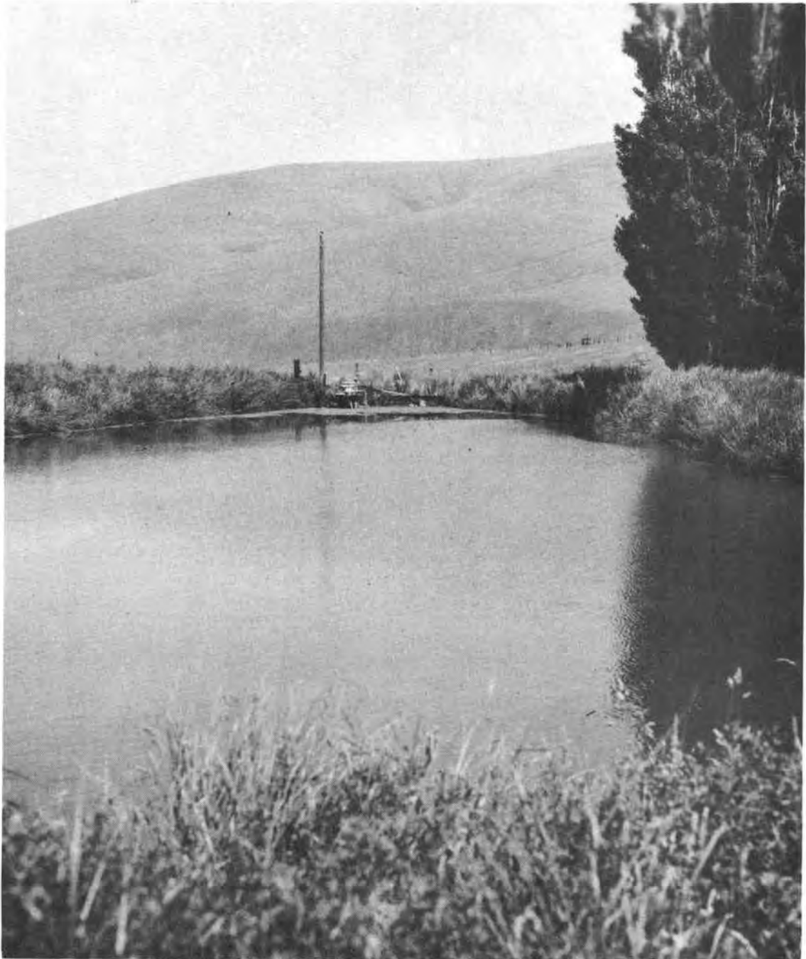
Figure 41.--A typical small reservoir constructed for multiple use in subbasin 3. SCS photo.
