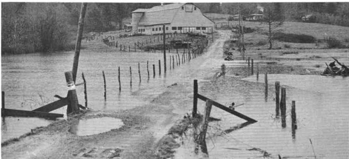
Photo 26.--This farm road near Cloverdale, Oregon, has been frequently damaged and closed by floods. SCS photo
