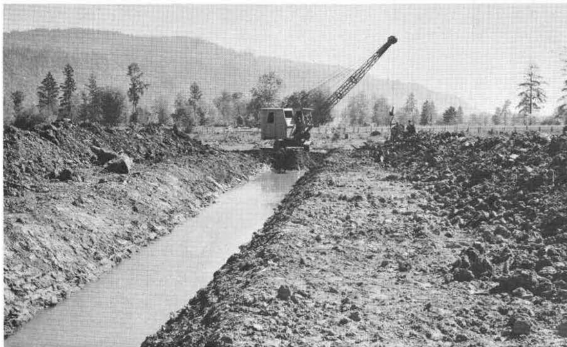
Photo 31.--Often tile cannot be used successfully to drain land until outlet ditches have been built, Tillamook County, Oregon. SCS photo
