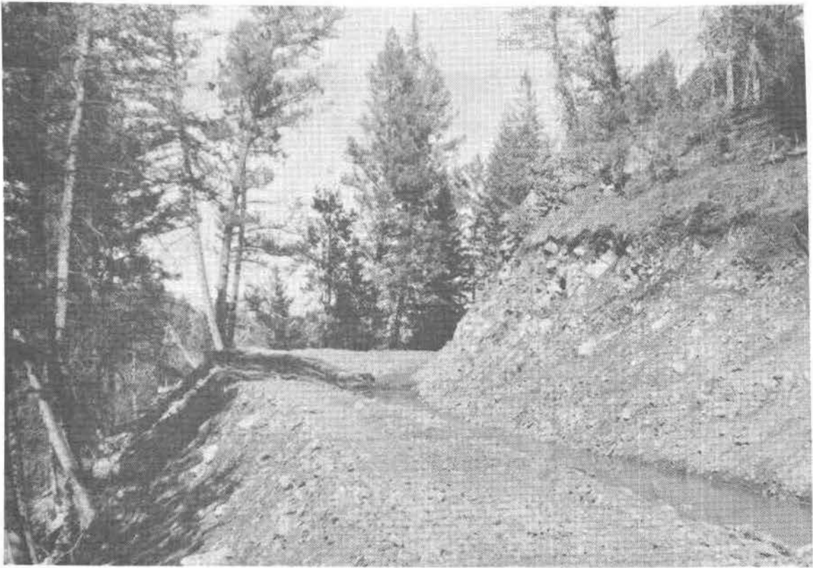
Photo 26.--This is a typical diversion for irrigation water in the Powder Drainage Basin.
