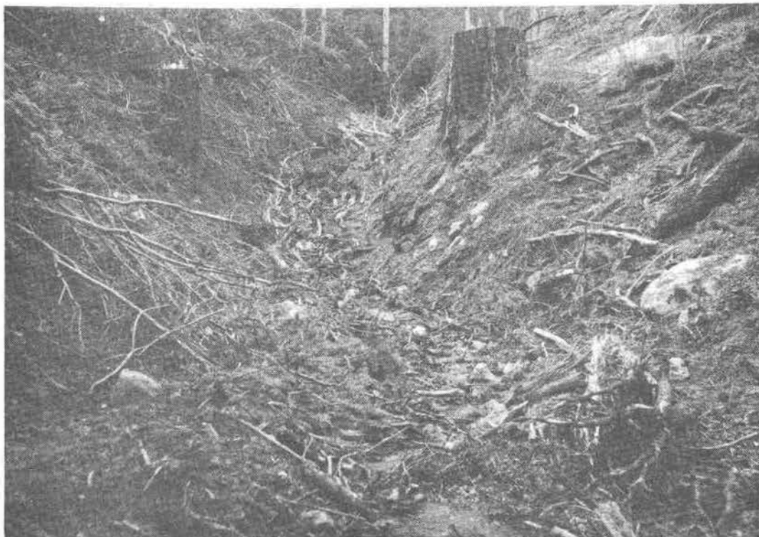
Photo 31.--Using a waterway for a downhill skid trail causes many problems. SCS
