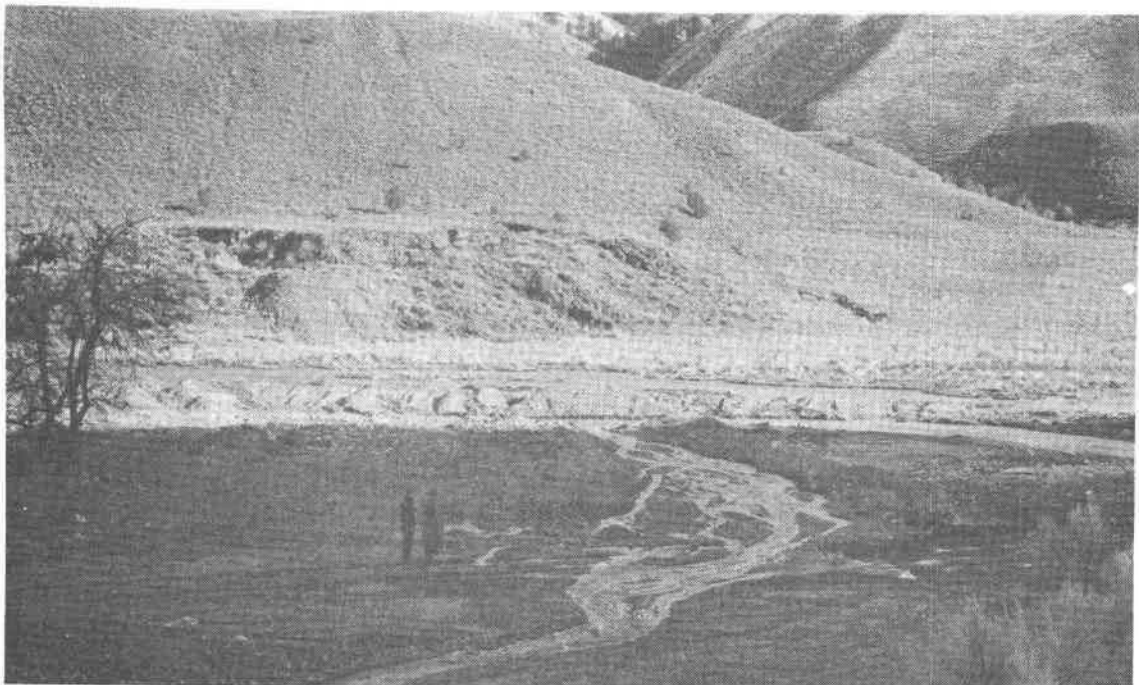
Photo 22.--A cloudburst caused the Burnt River near Bridgeport to overflow its banks resulting in erosion and flood damage.
