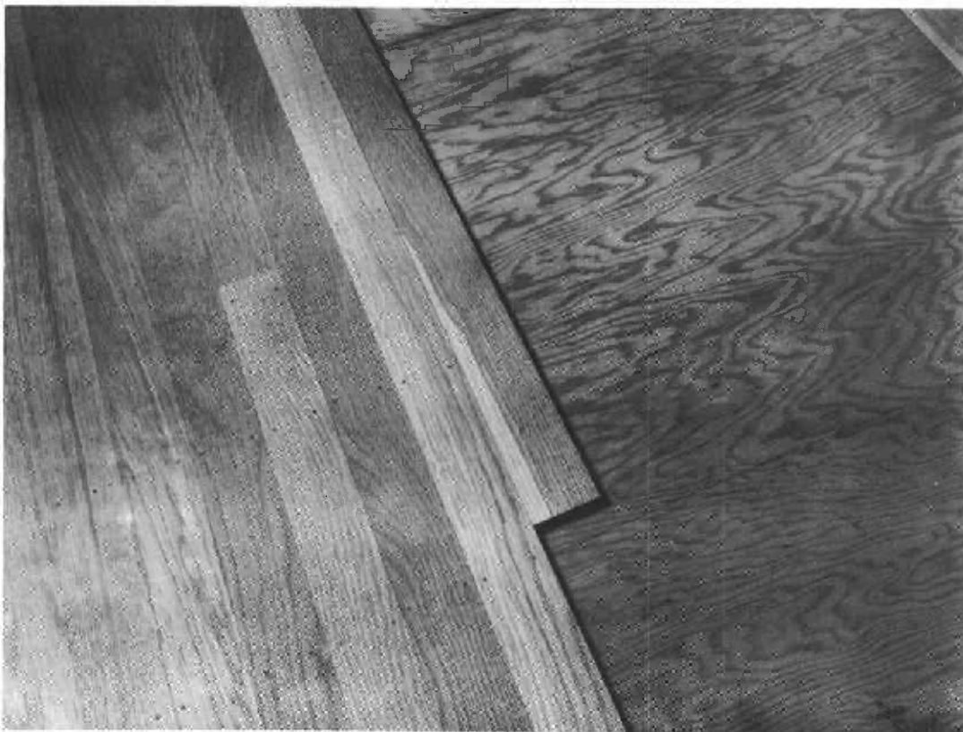
Figure 3. --Forest Products Laboratory office face-nailed, thin-strip white oak flooring during laying (March 5, 1951).
