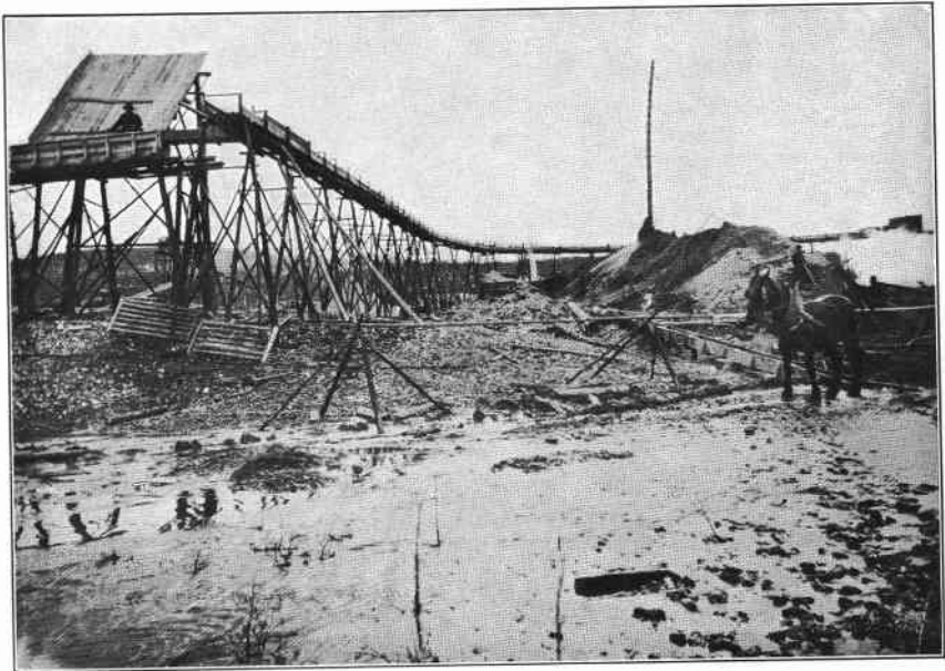
FIG. 2.—TYPICAL FLUME AND SLUICE BOXES USED IN PLACER MINING FOR GOLD IN THE FAIRBANKS DISTRICT. MUCH LUMBER AND MANY POLES ARE REQUIRED FOR THESE PURPOSES.
