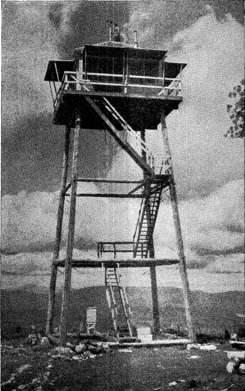
FIGURE 10.—Lookout-station exposure of three-cup anemometer, on roof, and of single-magnet register, inside cabin. (Elevation of station, 5,500 feet.)
