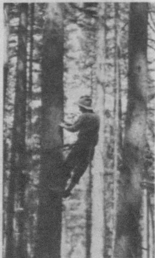
Repairing telephone line near Bumblebee Peak, Coeur d'Alene National Forest, 1932.
