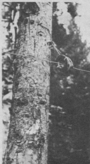
Split tree insulator holding telephone wire.
