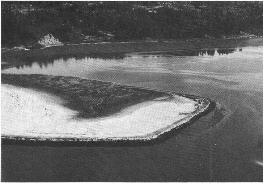
Figure 3. This tideland fill in Sallys Bend destroyed shellfish beds and altered current patterns in this area. Material eroded from the area covered stands of eelgrass and shellfish beds adjacent to the fill.
