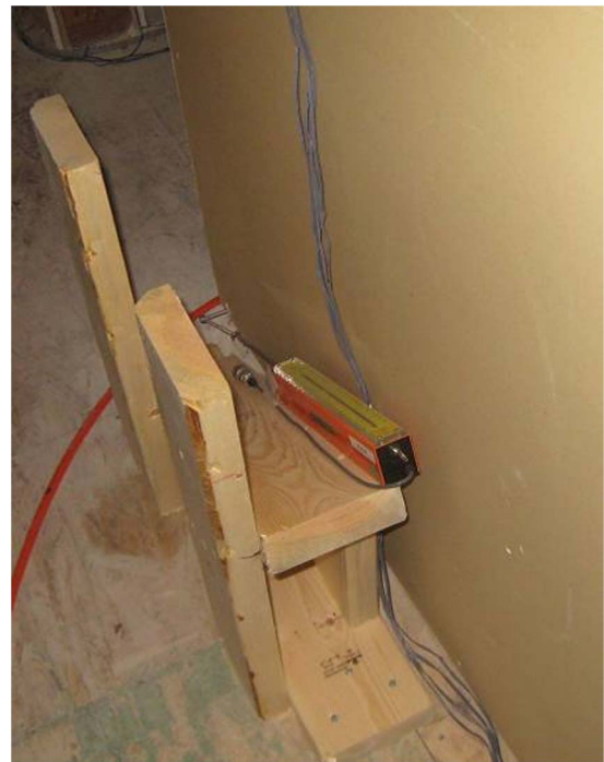
Fig. 3. Diagonal deformation measurements using stringpot
