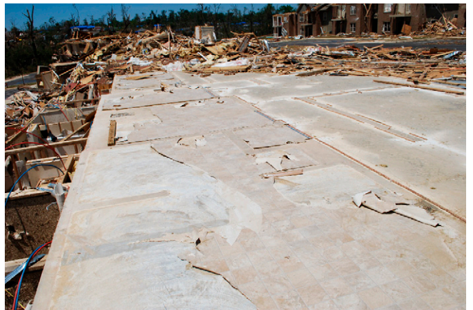
Fig. 13. Example of observed DOD10: newly constructed (2010) apartment complex with slab swept clean
