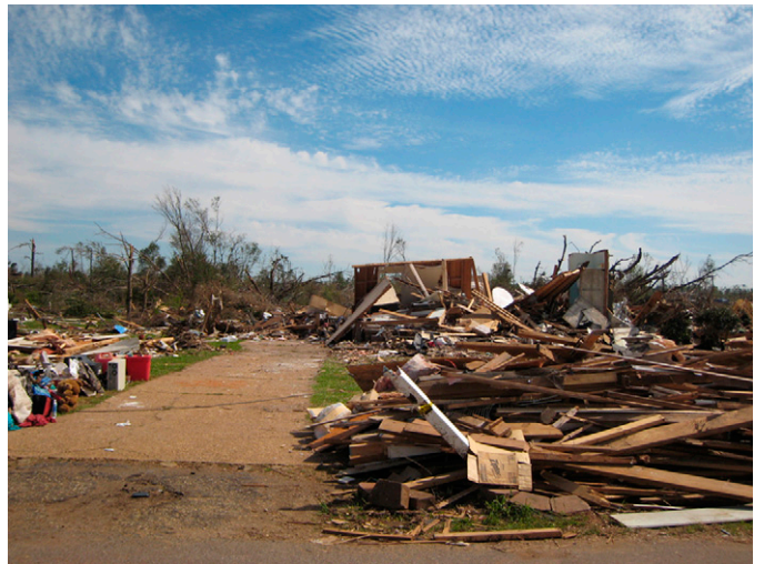
Fig. 12. Example of observed DOD8: most walls collapsed
