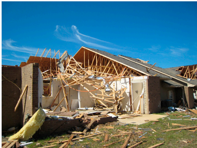
Fig. 10. Example of observed DOD6: large sections of roof removed
