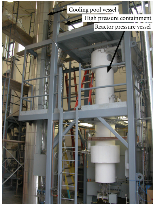
FIGURE 2: OSU-MASLWR experimental facility photo [1, 2, 13].
