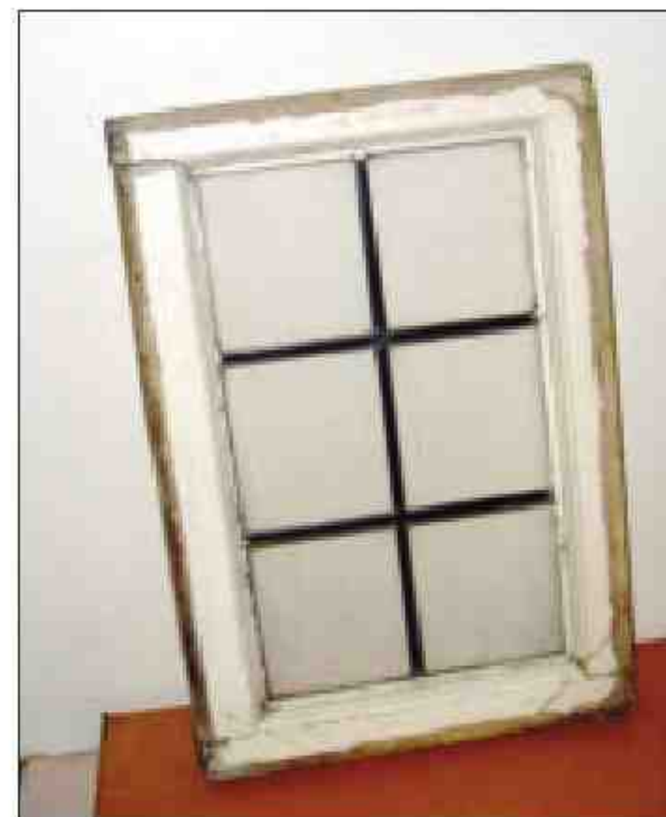
The frame of this window, which was purchased for $85.00 in an antiques store, is covered with chalky lead-based paint.
