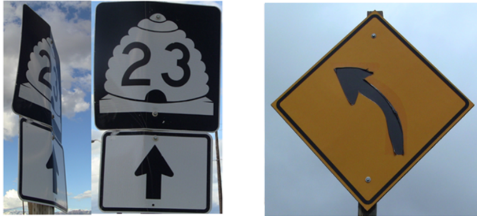
A. Bending Damage
