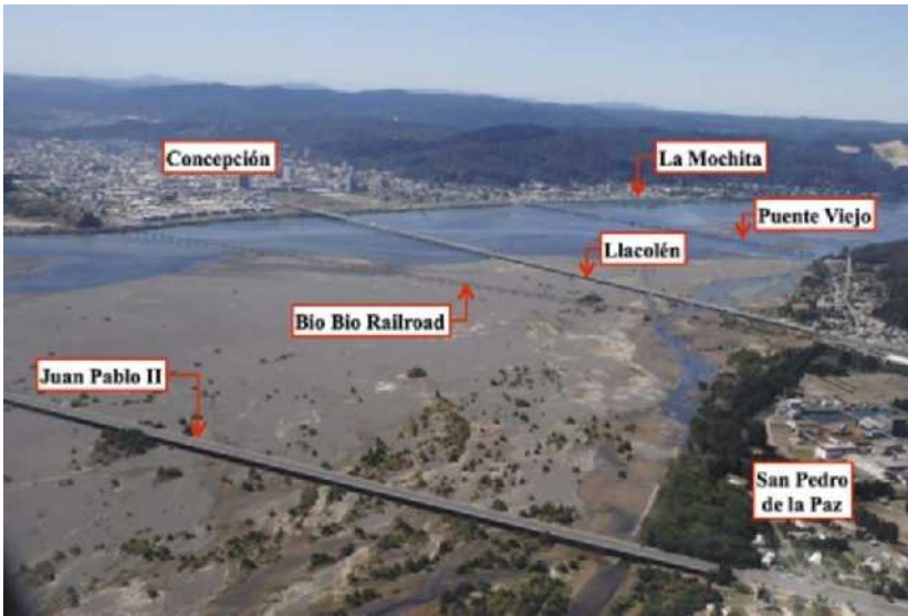
Figure 2. Aerial view of Concepción metropolitan area and Bio-Bío River main crossings.
