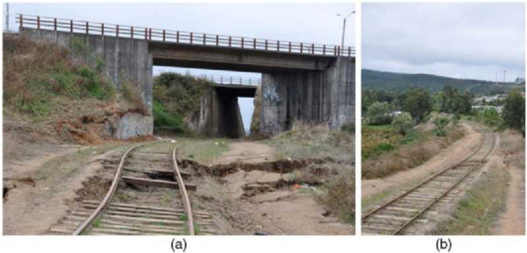
Figure 25. (a) Slab and girder-type overpasses at northern end of road embankment failure area, showing railroad and supporting ground settlement (view looking west), S37.0729° W73.1469°; and (b) ground failure below elevated railroad east of road embankment failure (view looking east), S37.0727° W73.1471°.
