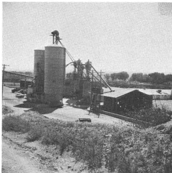
Concentrate storage, elevator arms, and feed mill structure of a feedlot producing more than 40,000 hundredweight of feedlot gain annually.
