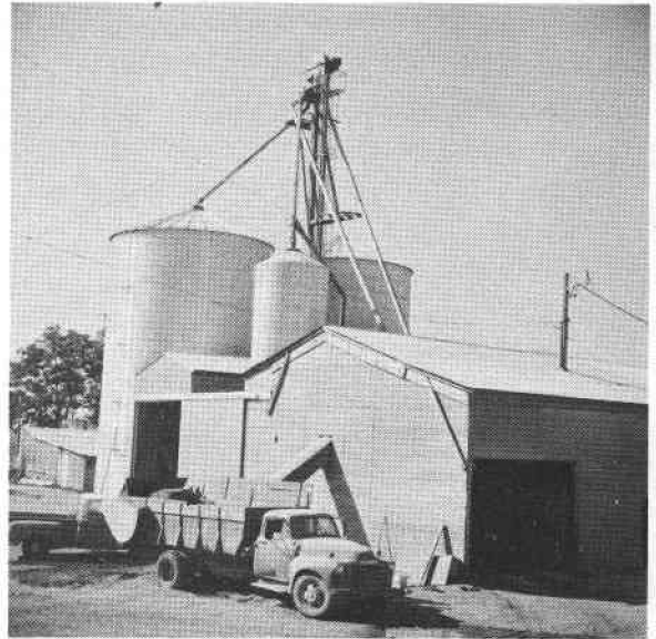
Concentrate storage bins, elevator arms, silage truck, and feed mill structure of a feedlot producing between 6,000 and 11,499 hundredweight of gain annually.
