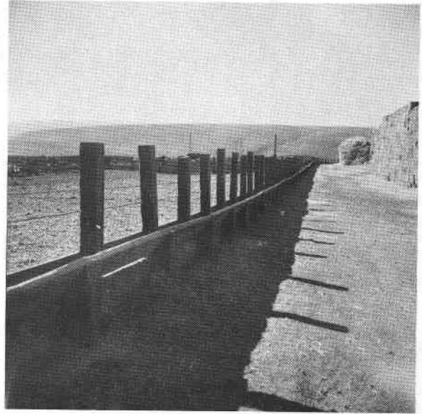
Fence-line bunk using "tie pipe", plank, and cable.
