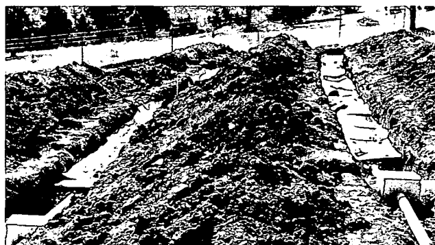
Figure 34.—Septic tank drainfield. A network of perforated pipes distributes sewage effluent evenly throughout the entire area of the drainfield. Each pipeline is surrounded by crushed rock, covered with paper, then covered with soil. This drainfield is on a slope, and pipelines are installed across the slope.
