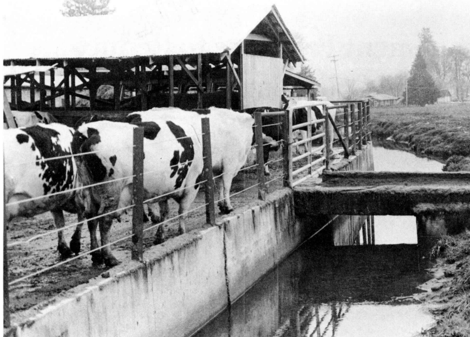
Figure 2.—A concrete holding area with a curb keeps the animal manure and rainwater from entering the adjacent stream. A curbed bridge allows the dairy operator to scrape the manure to a nearby storage area.
