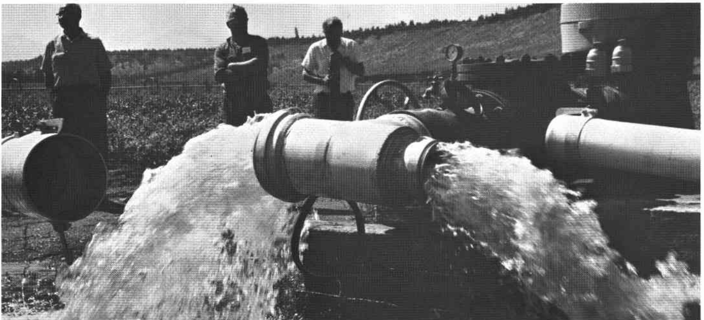
Development of underground sources of water for irrigation has taken place in the Lower Bridge area of the county during the last two years. Six wells, delivering 10,400 gallons of water per minute, are now in use. Depth varies from 140 to 300 feet and the amount of water delivered from 500 to 3,500 gallons per minute. About 1,800 acres of land have been brought under irrigation and supplemental water has been furnished for 700 acres. (Photo by M. L. Myrick, Redmond Spokesman)
