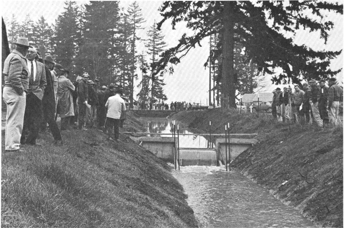
Water resources of Yamhill Co. must be developed to the fullest extent. An outstanding example of community cooperation is the development of the Palmer Creek pumping station.
