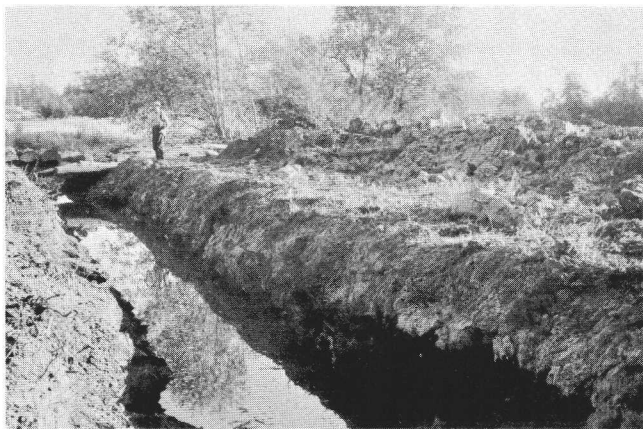
Open Ditches Provide Necessary Drainage to Diked Farmlands
