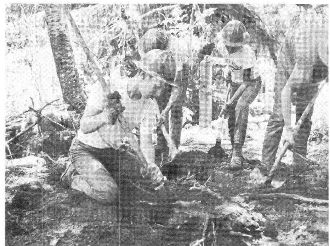
Summer Youth Workers Build County Parks
