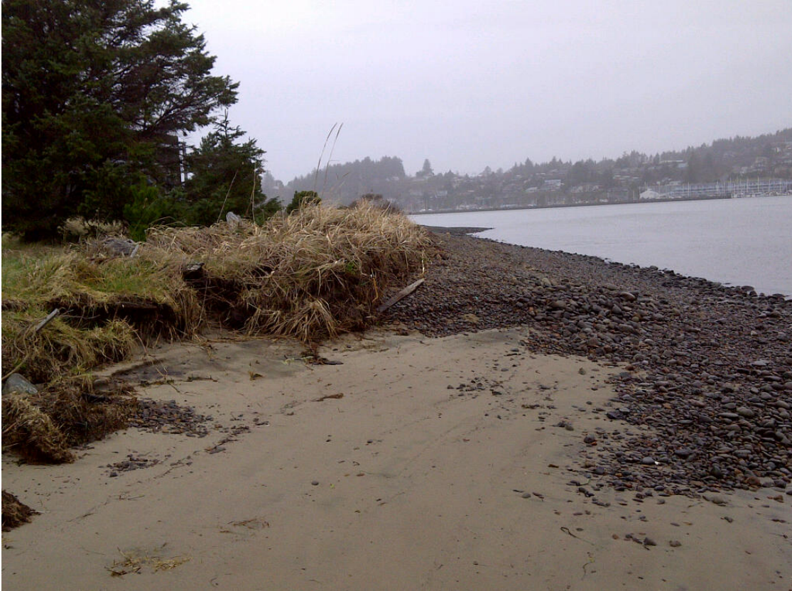
Figure 4.5: View of the southern end of the 2011 DRP (February 14, 2014). Erosion has removed high salt marsh vegetation and is beginning to erode shoreline protected by the DRP.
