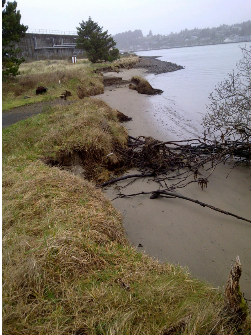
Figure 4.3: View of eroded section of HMSC nature trail, February 14, 2014. The trail has been completely washed out in the section shown in Figure 4.2, and collapsed asphalt has been removed. Another of the Reference area monitoring quadrats for the vegetation studies (PVC stake in center of picture) has been lost to erosion.
