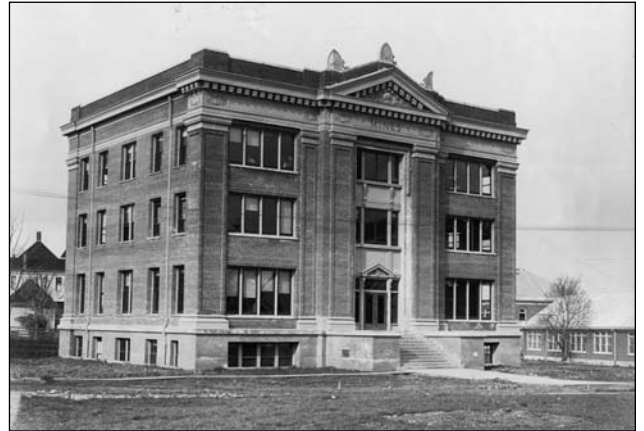
Mines Building, 1913–1940; renamed Batcheller Hall to honor mining engineering professor (see page 3) .
