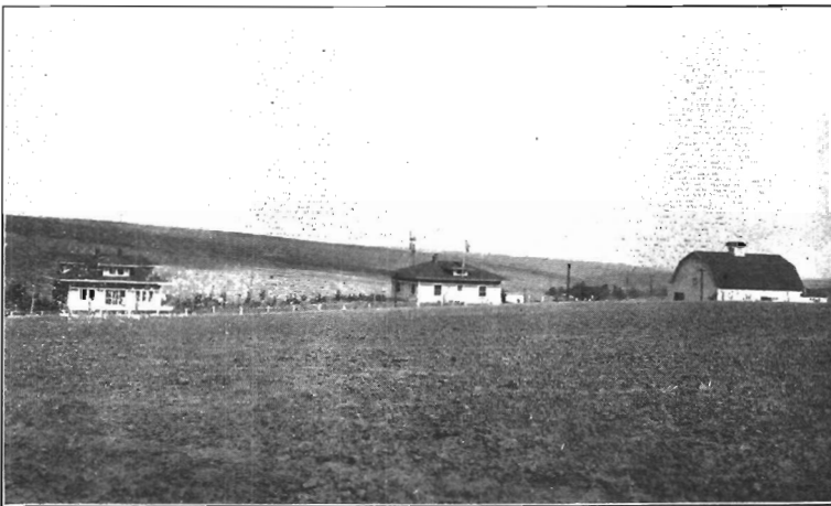
Fig. 2. General view of the Station buildings.
