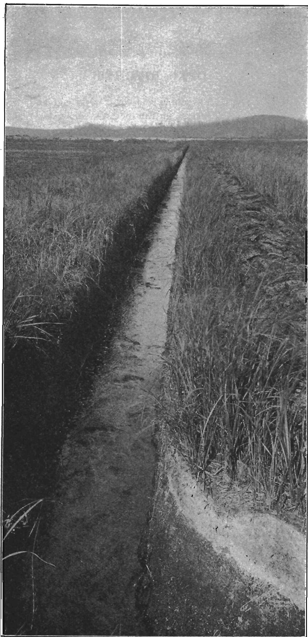
Figure 36. Open Lateral in Peat—Clatskanie.
