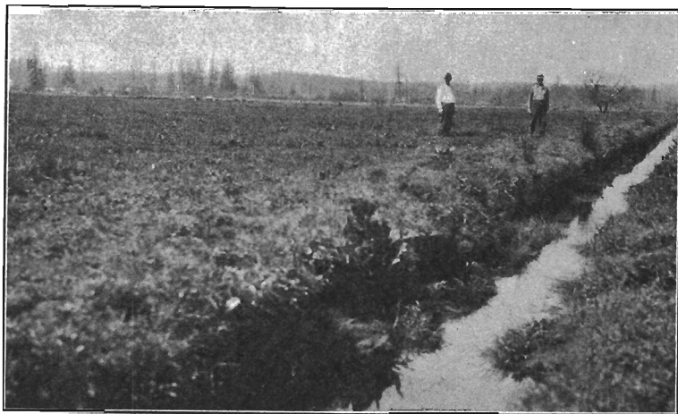
Figure 31. View of Tillamook Drainage District Showing Waterlogging Before the Old Ditch was Deepened and Enlarged.
