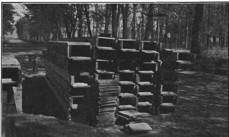
Figure 14. Box Drains—Mallet, Oregon.
