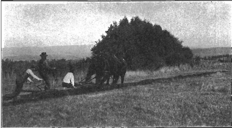
Figure 19. Starting a Ditch in Tough Sod.
