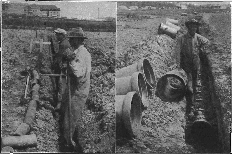
Figure 23. Finishing Trench and Laying Tile, Oregon Experiment Station.
