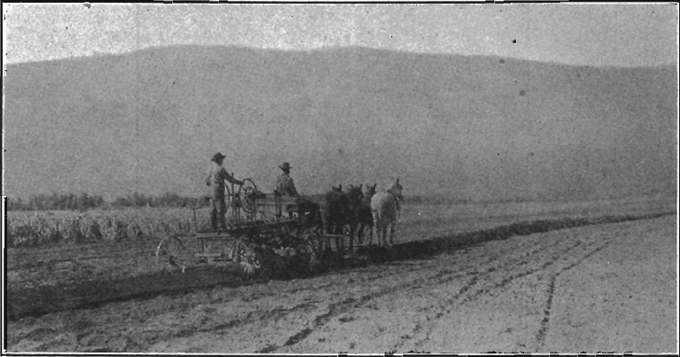
Figure 26. Filling Tile Ditch with a Light Road Grader.
