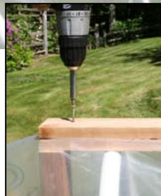
Figure 9 insert. Secure the plastic with 1.5-inch screws.
