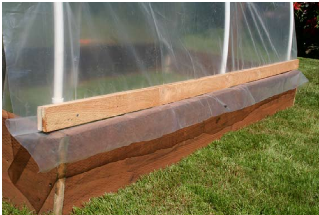
Figure 10. Secure the side curtain plastic with two D boards that sandwich the plastic and rest on top of the raised bed. Trim excess plastic, but leave 6 to 8 inches of overhang.
