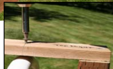
Figure 5 insert. Secure the backbone to the C board and the rib.
