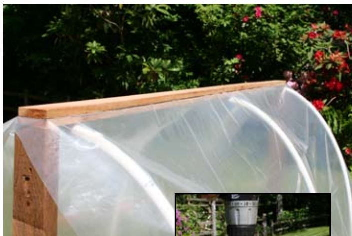
Figure 9. Sandwich and secure 10 x 10-foot plastic between the two D boards.
