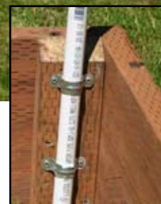
Figure 4 insert. Insert pipe straps.
