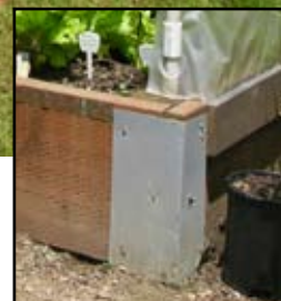
Figure 3 insert. Outside corner metal straps add stability to the raised-bed base.
