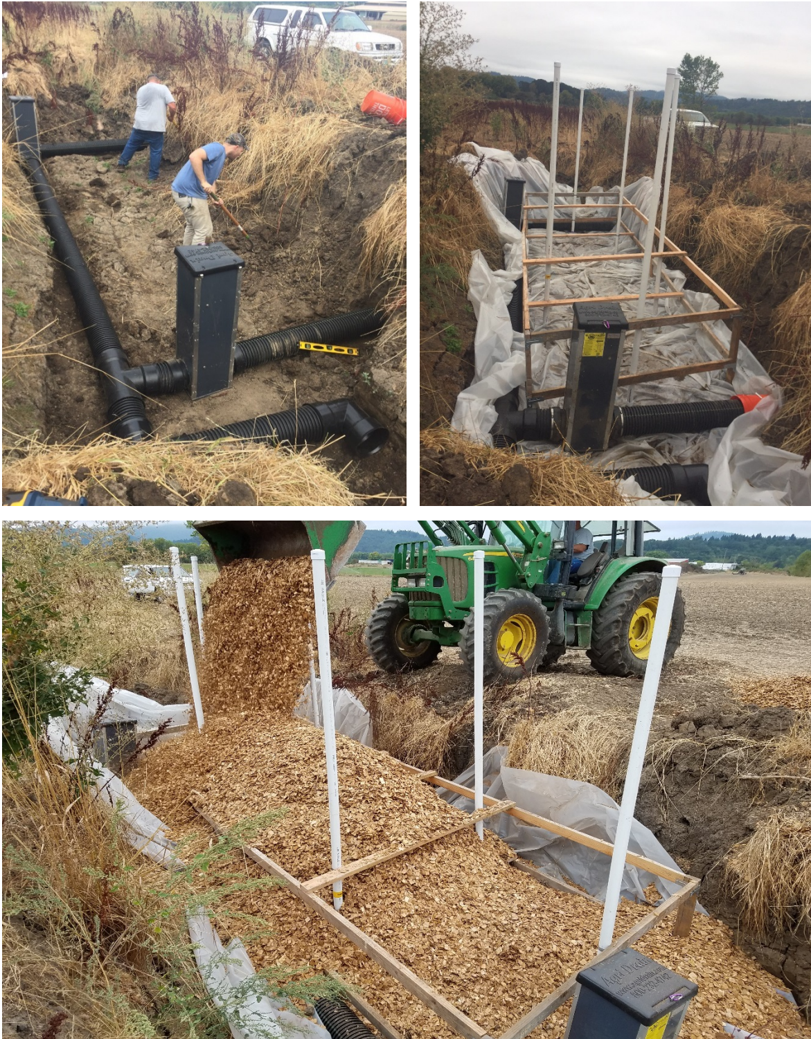
Figure 3.3: The construction process of the denitrifying bioreactor evaluated in this study
