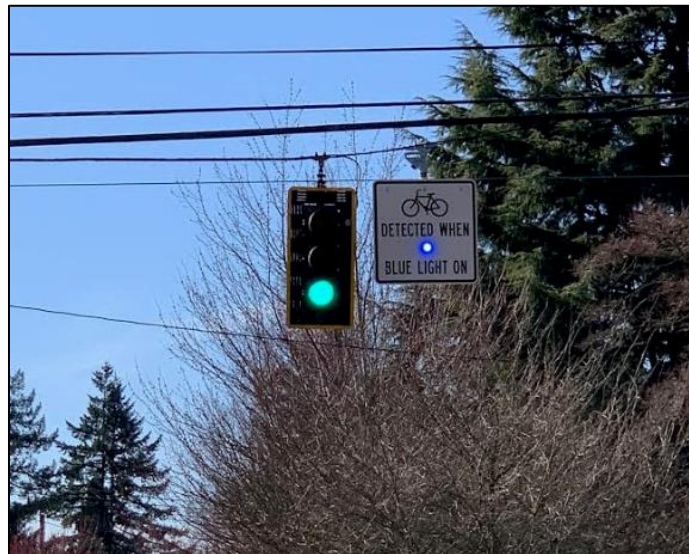
Figure 2.11 BLDF in Traffic Signal Housing with Accompanying Sign
