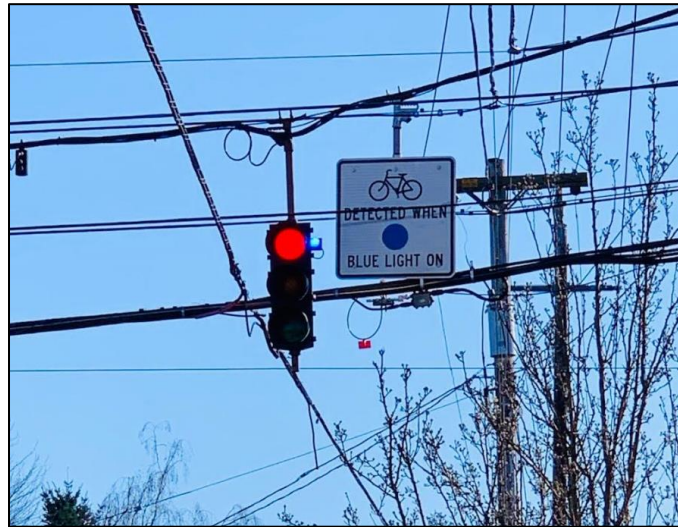
Figure 2.11 BLDF in Traffic Signal Housing with Accompanying Sign
