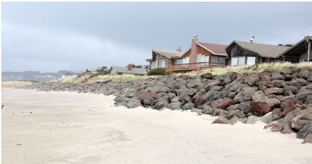
Riprap in Neskowin, OR
