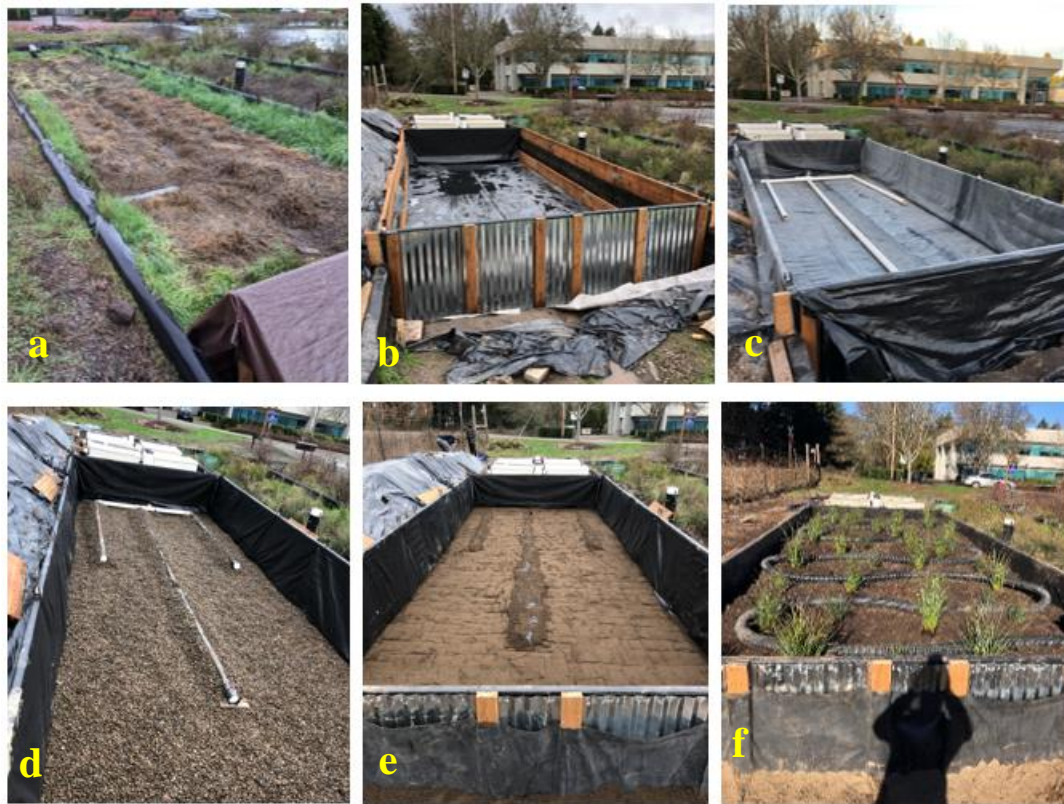
Figure 3.4 Progress photos taken during construction of the LID. (a) Cell 1 before excavation. (b) Completed LID frame. (c) Installation of pond liner and underdrain. (d) River rock layer. (e) Compacted sand layer. (f) OGSIR soil with perforated hose, native vegetation, and mulch.
