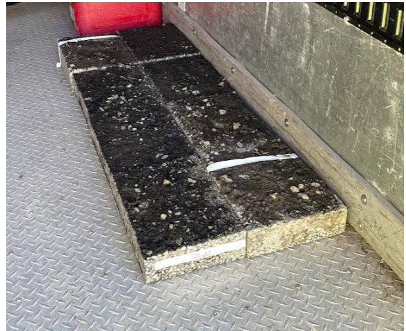
(j) Typical asphalt blocks extracted from the test section
