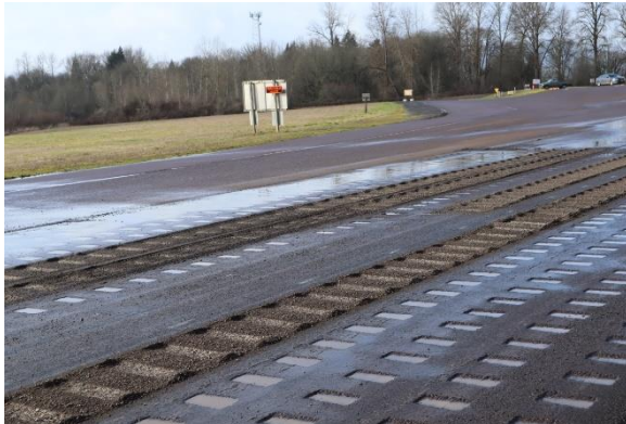
(e) Section during CLRS milling (2/26/2021)
