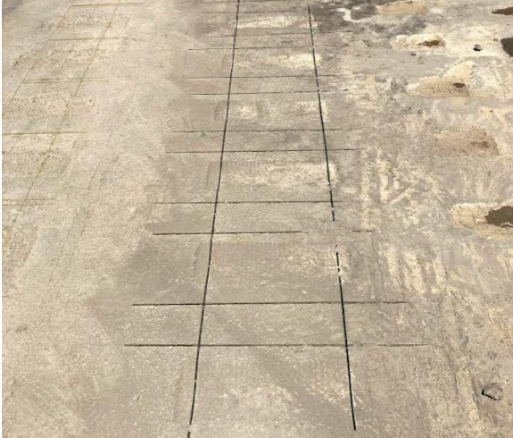
(i) Typical asphalt slab cuts using the walk-behind saw
