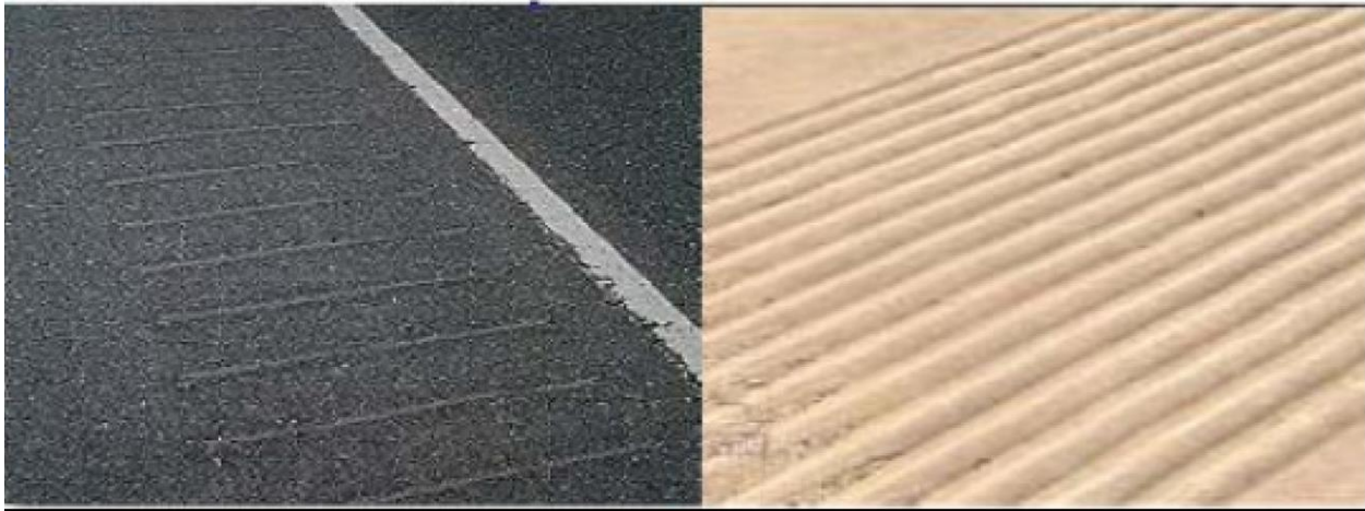
Figure 2.4: Rolled or formed rumble strips (Richards and Saito, 2007) (Guin et al., 2014)
