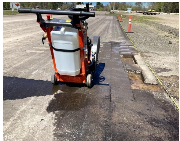
(h) Diamond blade walk-behind saw
