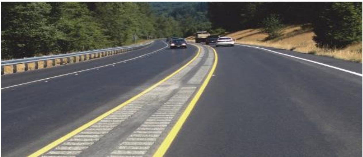
Figure 2.1: Example of a centerline rumble strip on asphalt pavement (National Academies of Sciences, Engineering, and Medicine, 2016)
