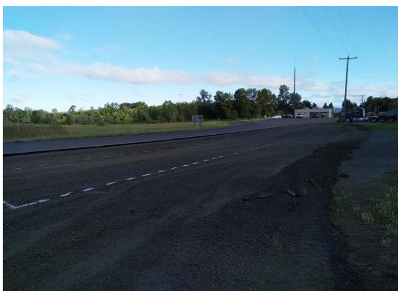
(a) Section before construction (6/25/2020 – 7am)
