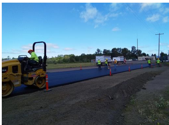
(b) Section construction (6/25/2020 – 12pm)
