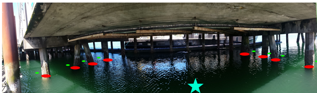
Figure 3.6: Oregon State University Ship Operations Pier in Newport, Oregon used for field trials. The robot must visit each of the inspection locations indicated by green dots while avoiding becoming entangled by the wharf pilings shown as red circles. The robot is deployed from the base station located at the blue star.
