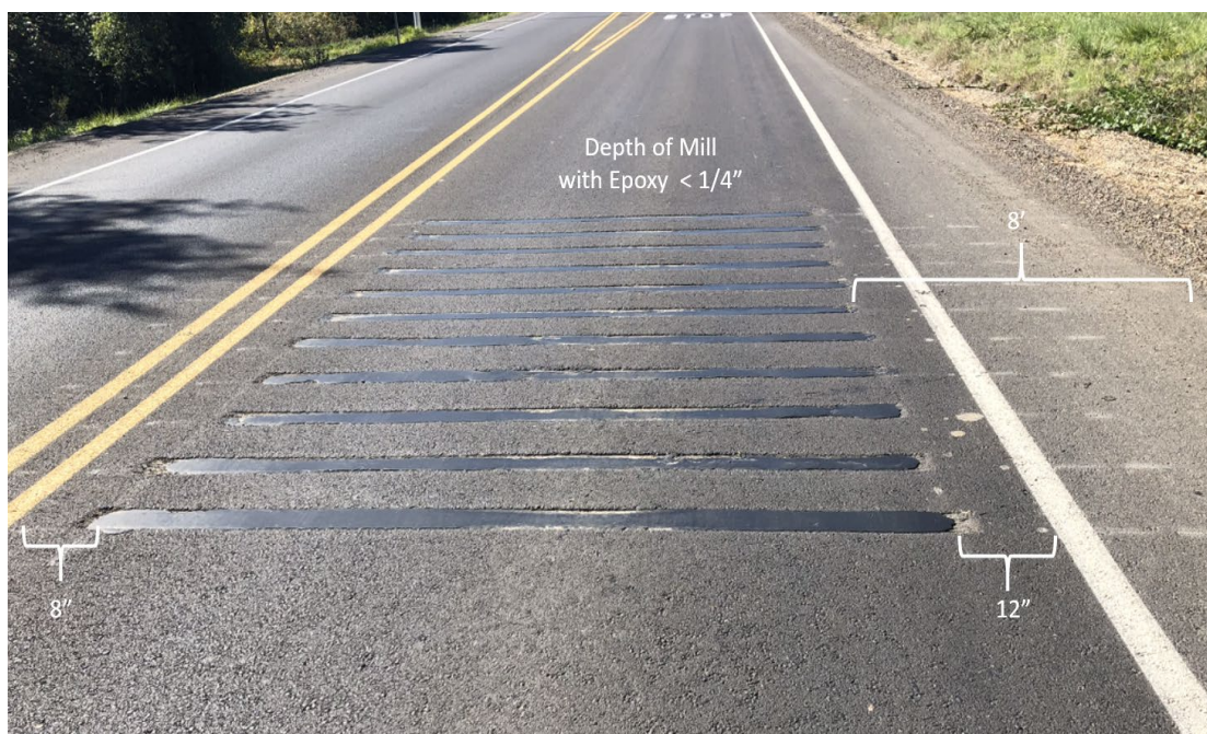
Figure 4.4 After condition: Epoxy filled TRS at near location
