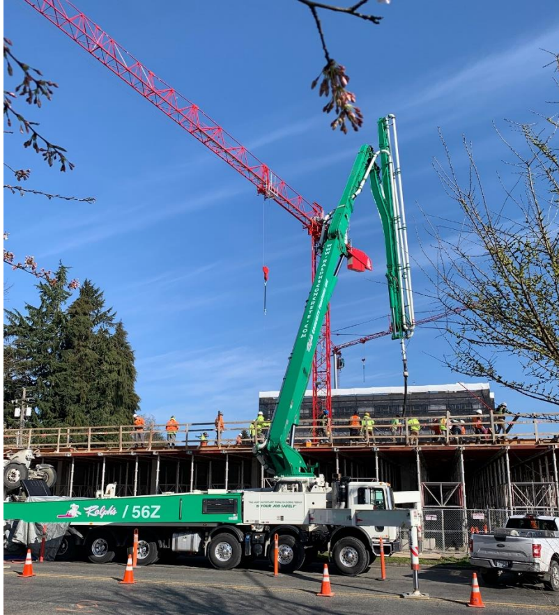
Figure 4.21. Concrete Placement in Progress
