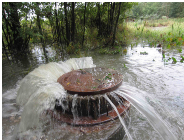
Fig. 1. Sanitary sewage overflow in Columbia, SC (Location 5E in this study; photo: S. Rothenberg).
