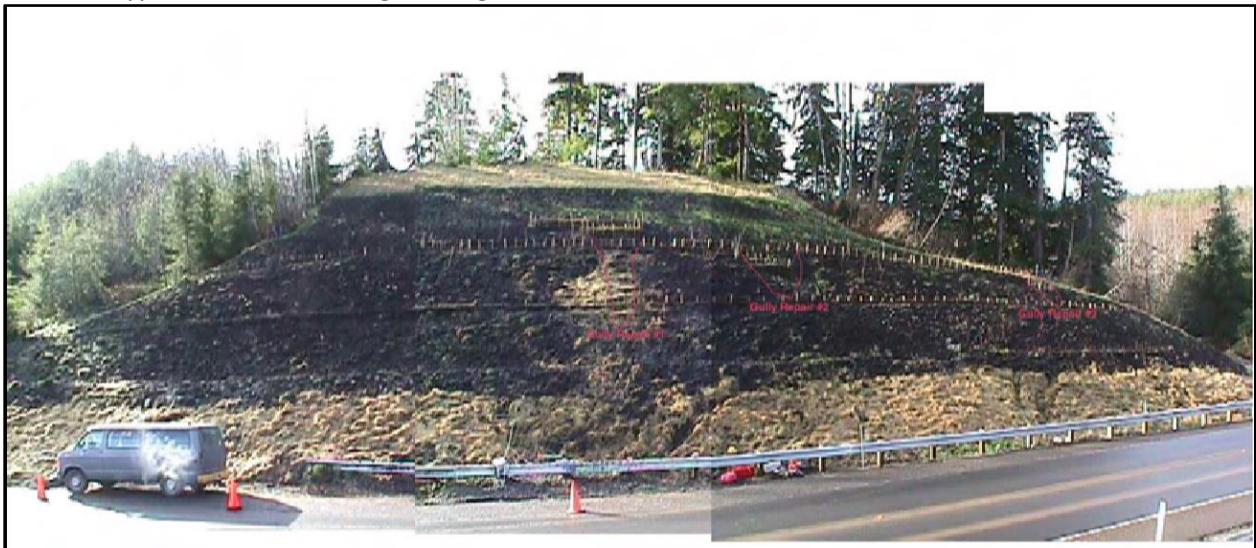
Photo 6. Typical roadside bioengineering work.
