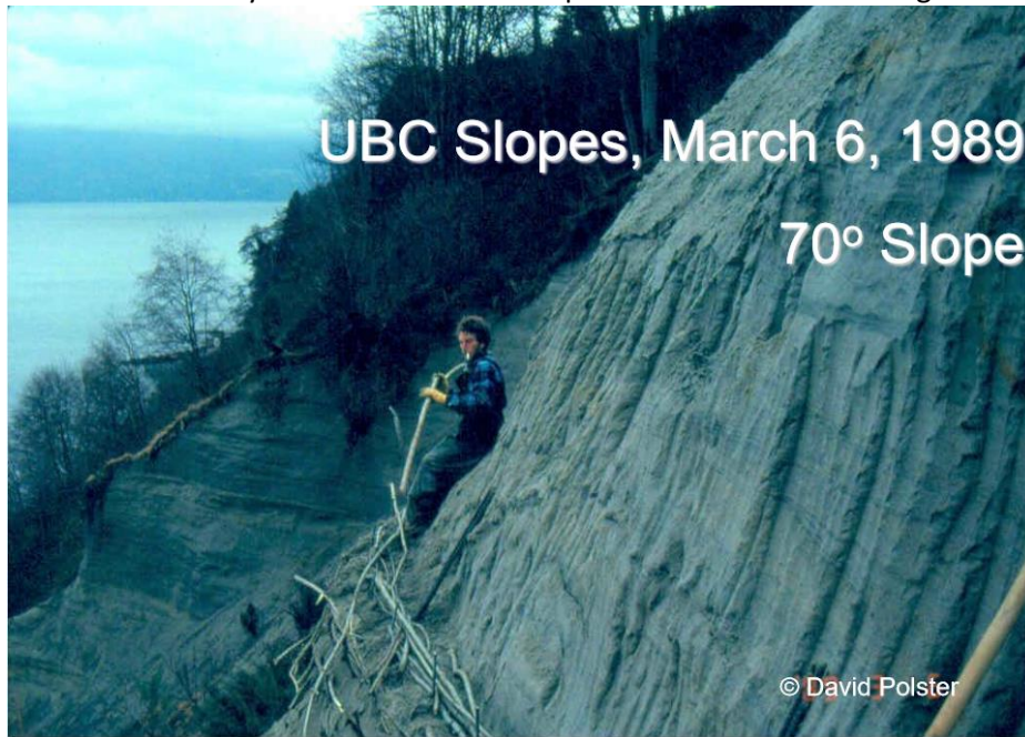
Photo 7. University of British Columbia slope stabilization work during construction.
