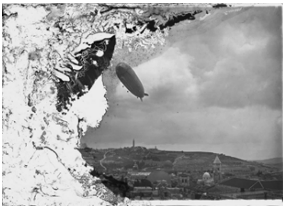
Emulsion has peeled away from the base
