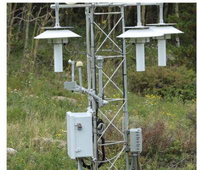
Three Aspirated and solar shielded temperature sensors adjacent to sDFIR at C1. Anemometer in the background on boom.
