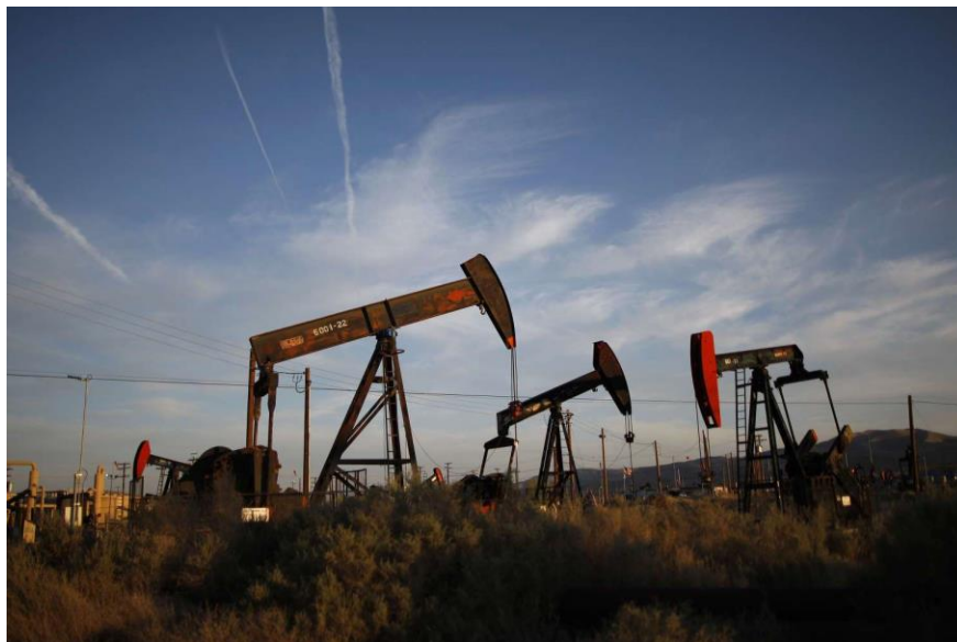
Figure 7: Hydraulic fracturing systems can often be seen just off of main roads.
