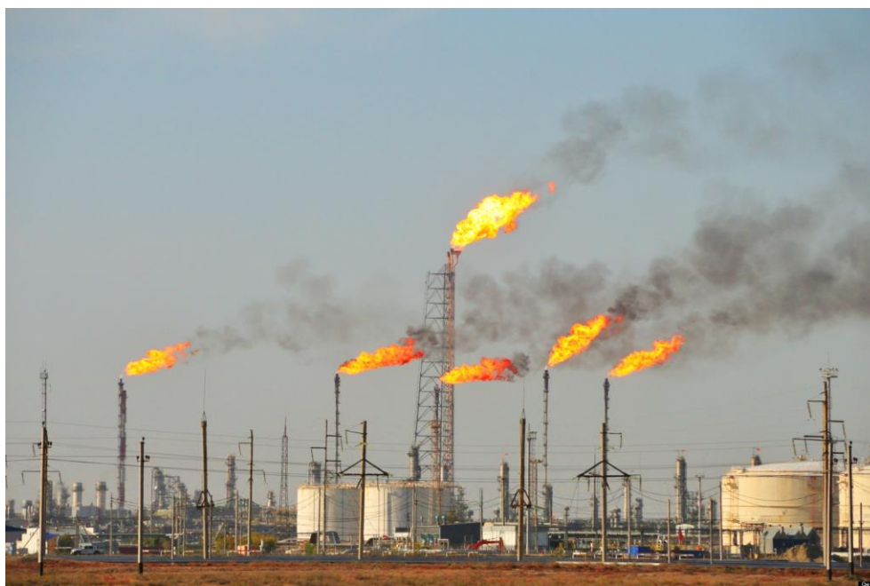
Figure 8: Flares from Natural Gas and Oil Refinery
